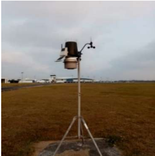
Figure 5 Anemometer installed inside the runway area
