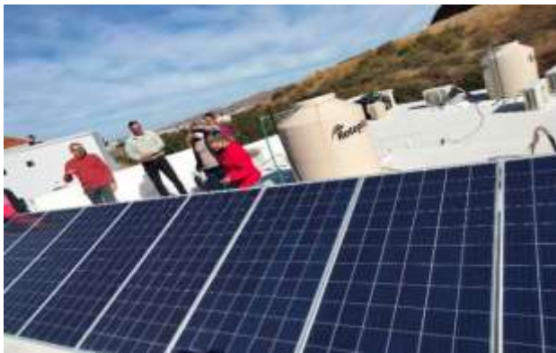
Figure 8 Physical installation of the FVSS, Case 1
