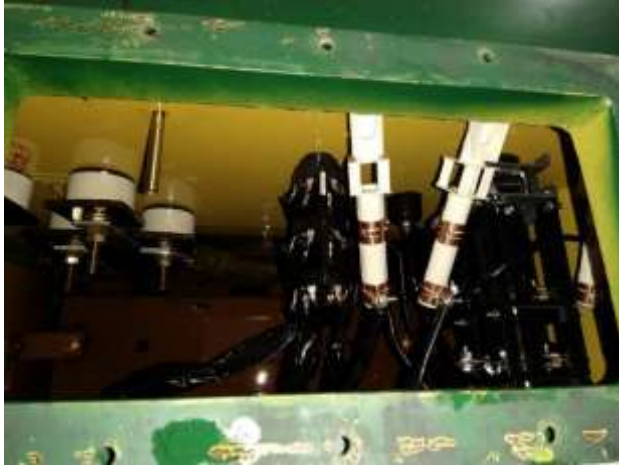
Figure 1 75 kVA pad-mounted transformer insulation system
