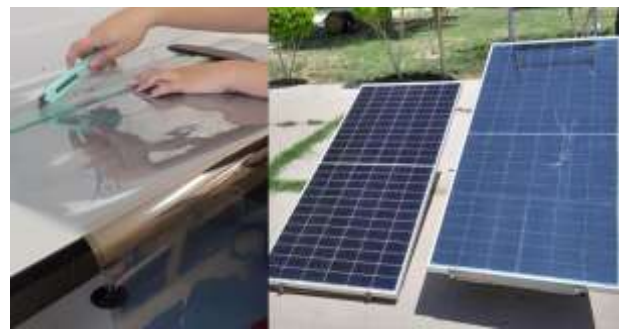
Figure 6 Installation of nano-ceramic film in photovoltaic module Own Elaboration
