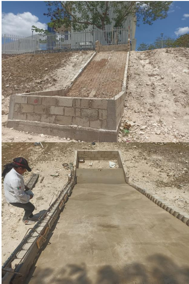
Figure 5 Screen construction. a) Laying of electro-welded mesh, b) Casting Source: own elaboration
