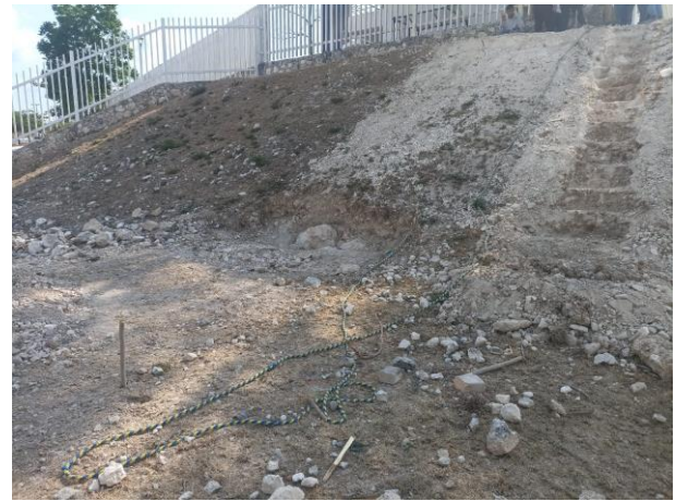
Figure 2 Trace and leveling of the land Source: Own elaboration
