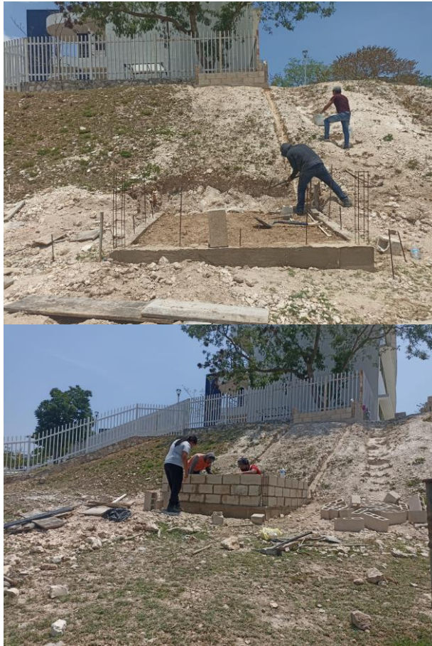
Figure 4 Bottom tank construction. a) Foundation, b) Construction of walls
