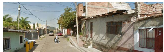
Figure 7 Road and houses damaged by a settlement in Jocotepec (Photograph from the Maciel-Flores archive). Guadalajara - Colima Highway (Mex. 54), kilometer 6 approximately, there is a constant settlement near the intersection with the railroad
