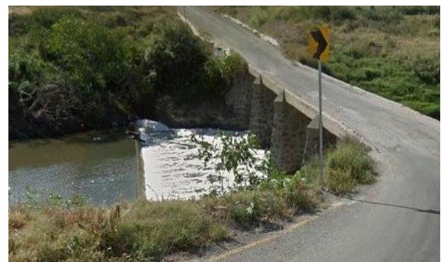
Figure 6 Bridge Source: (Google Earth) Simulations
