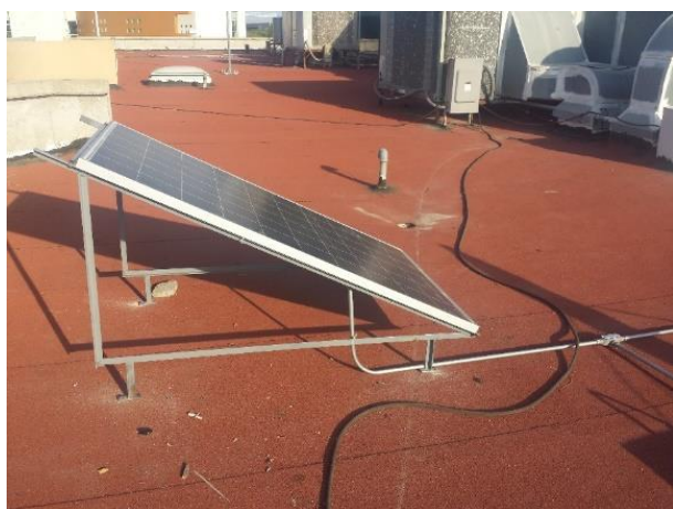
Figure 5 Panel with anchored support Source: Own elaboration
