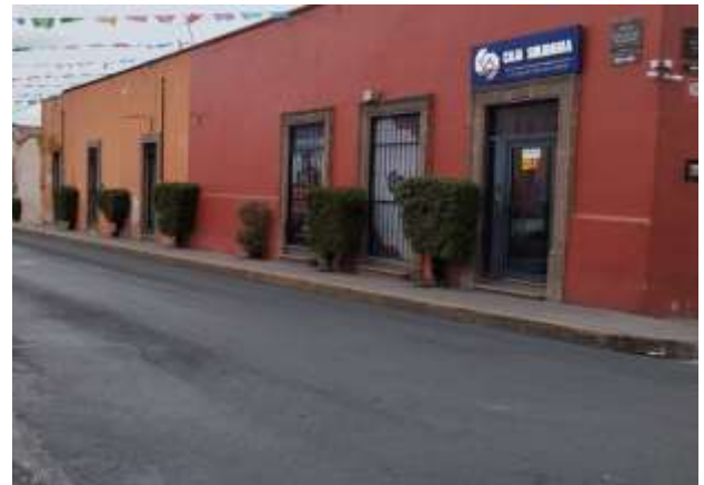
Figure 7 Facades of Huichapan Source: Project archive, 2023
