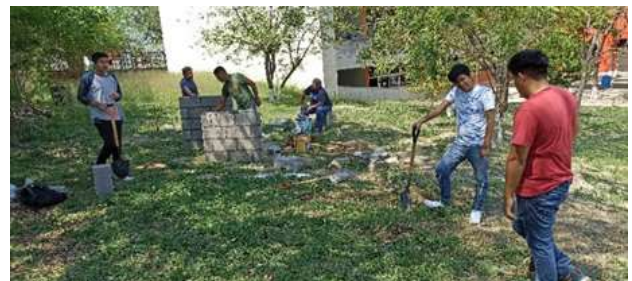
Figure 1 Wall construction Source: Own Elaboration
