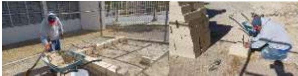
Figure 5 and 6 Placement of CEB-PET by skilled labor, 2023
