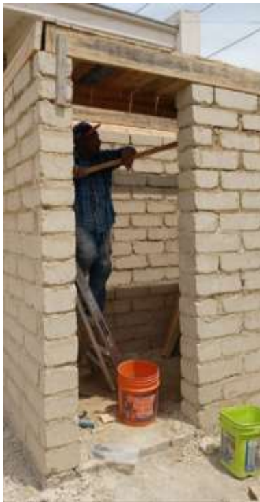
Figure 7 CEB-PET module developed by skilled labor, 2023
