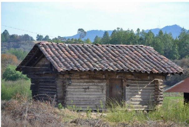
Figure 5 Rural vernacular wooden dwelling with morillos, no windows, wooden door frames with wooden beams and half-round roof tiles Source: (Hernández, 2018)
