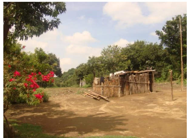
Figure 6 Vernacular dwelling with reed walls and roof in Tochimilco, Puebla Source: (Vázquez, 2018)
