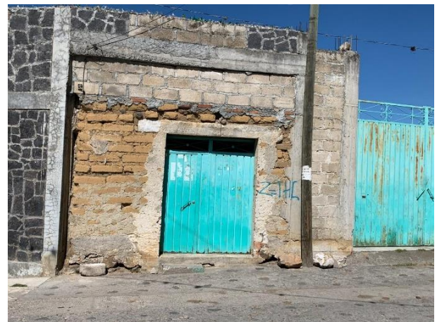
Figure 1 Vernacular dwelling of adobe, stone, block with concrete frames in Tochimilco, Puebla Source: (Vázquez, 2019)
