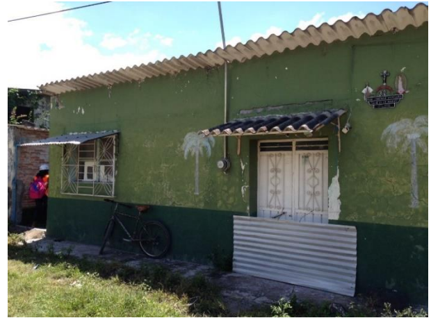
Figure 8 Vernacular dwelling with adobe walls and tin roofs in Chietla, Puebla Source: (Garate, 2017)
