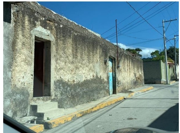
Figure 4 Vernacular house with concrete frames and cement cladding in Tochimilco, Puebla Source: (Vázquez, 2019)
