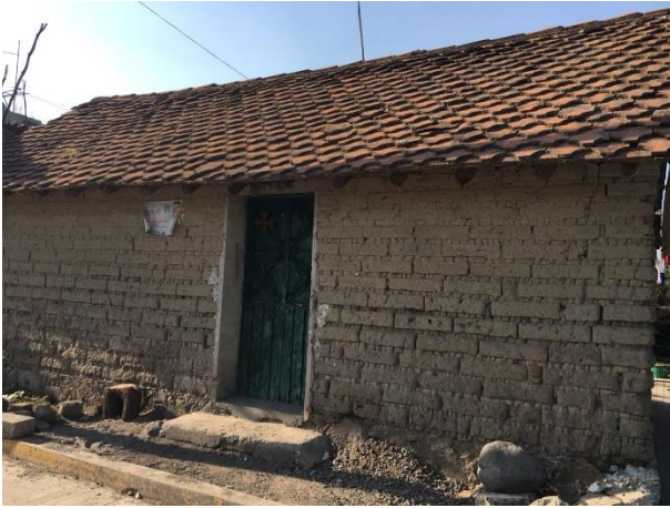
Figure 10 Adobe wall and prefabricated clay tile roof in Tochimilco, Puebla Source: (Vázquez, 2019)
