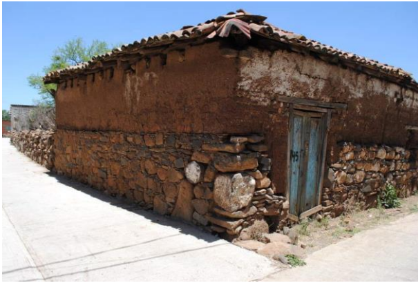
Figure 5 Vernacular housing of stone walls, adobe and ceilings of wooden beams and tile Source: (GARATE, 2016)
