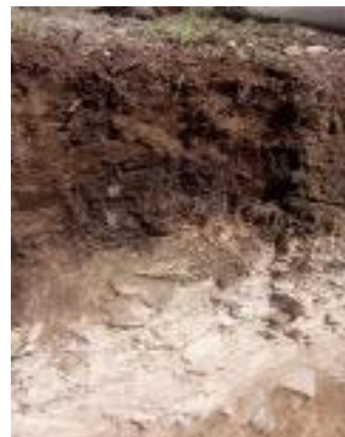
Figure 7 View of the walls of the open pit exploration well Source: Own authorship
