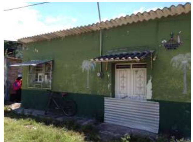
Figure 3 Adobe house in Chietla, the epicenter of the 2017 earthquake that was not affected, due to its construction quality. Buap, 2017
