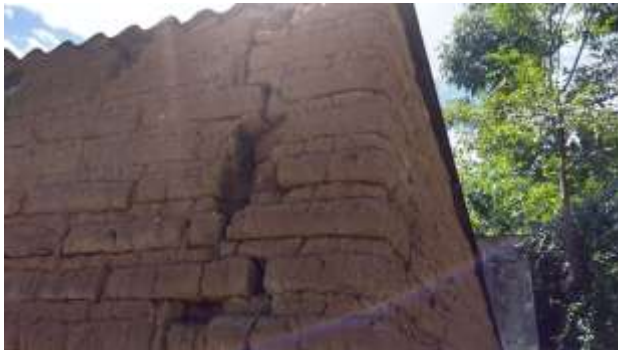
Figure 10 Housing in the neighborhood of San Juan Bautista, affected by the earthquake of September 19, 2017. Tochimilco, Puebla, 2017
