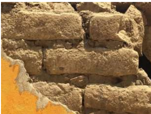
Figure 11 Clay mortar that joins the adobe in a historic building. Tochimilco, Puebla, 2017
