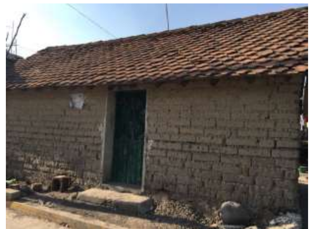
Figure 3 Adobe house that was not affected, due to its construction quality. Huaquechula, Puebla, 2017
