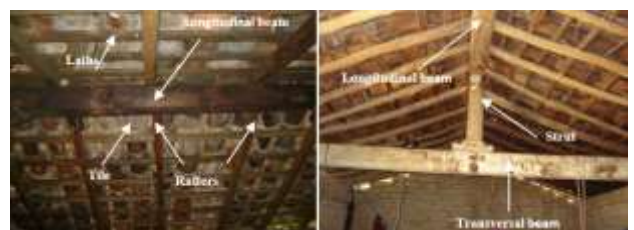
Figure 2 Roof system in adobe houses Self-authorship
