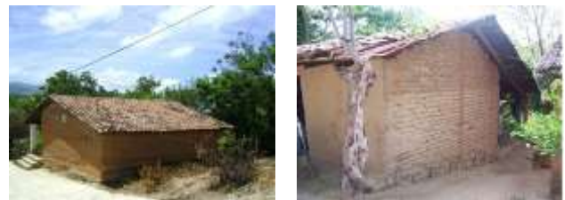
Figure 1 Typical adobe houses in Mexico Self-Authorship
