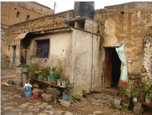
Figure 9 This image shows the adobe construction, divided into parts and each section is inhabited by a family and a room that is used for the toilet is attached to it Source: Vázquez, 2017
