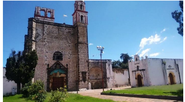
Figure 6 The cover of the church of the Assumption of Our Lady; to the right and next to the tower you can see the open chapel
