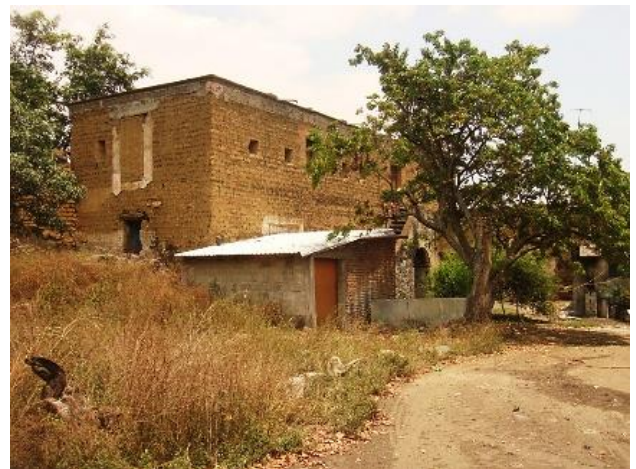
Figure 11 The back construction is of two levels made with adobe and in front is a new house that preserves the traditional characteristics of the vernacular house that they are. Rectangular shape and sloping roof Source: Vázquez, 2017
