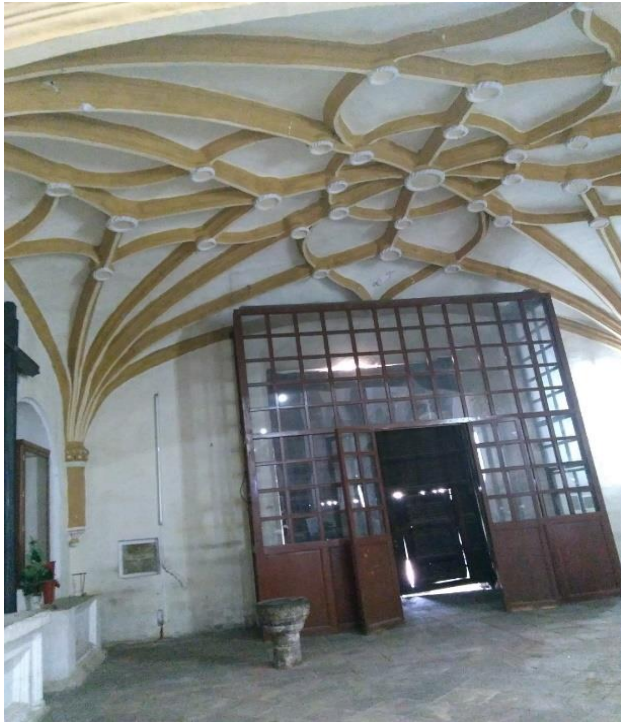
Figure 4 Inside the church where you can see the ribs of the ceiling where the choir is located
