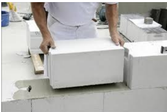
Figure 13 Tongue and groove block
