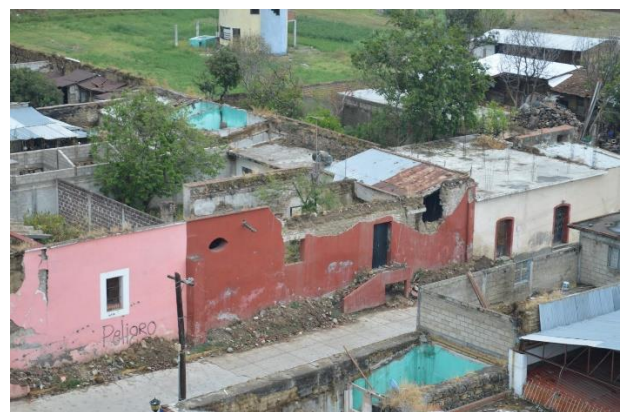
Figure 7 Aerial view of historic dwellings damaged by the earthquake of September 19, 2017 Source: Vázquez, August 2018
