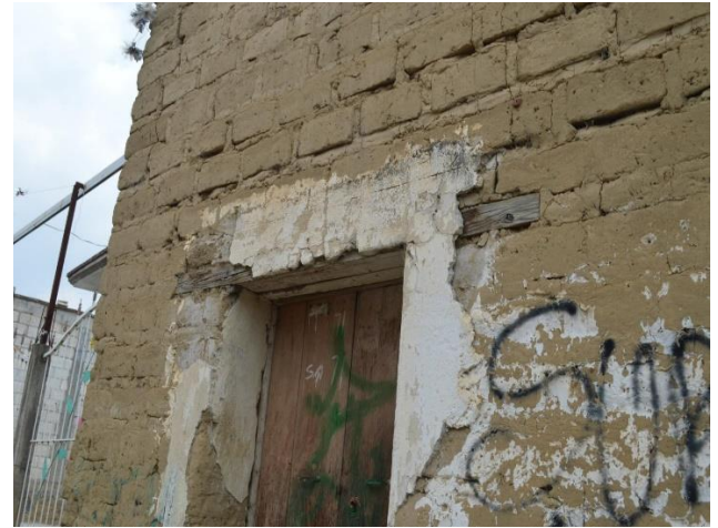
Figure 6 Vernacular dwellings without windows and with rectangular door Source: Vázquez, August 2018
