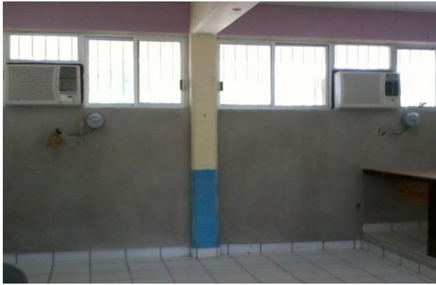
Figure 3 Meters provided by CFE for measuring energy consumption Source: UV FIME - Poza Rica
