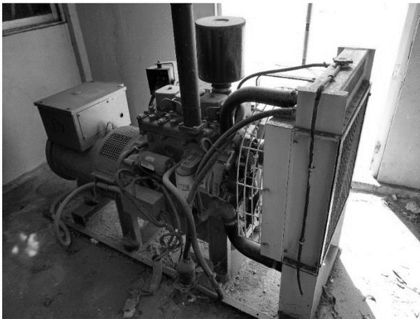
**Figure 3** Emergency electric generator of the clinic, operated with diesel
