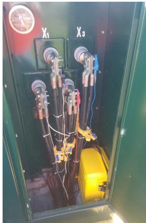
Figura 2 Three-phase HIOKI connection
