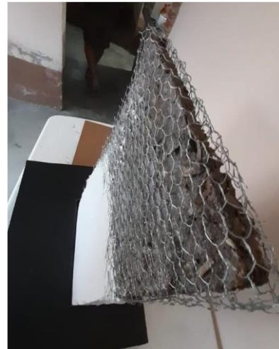
Figure 20 The figure shows the mesh that not only acts structurally, but also as a connection between panels
