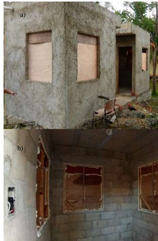
Figure 3 Building prototypes sealed with polyurethane expandable foam. a) Exterior, b) Interior
