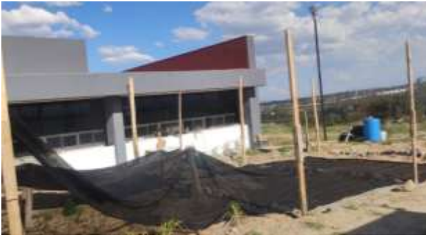
Figure 3 Placement of the posts for positioning the shade mesh
