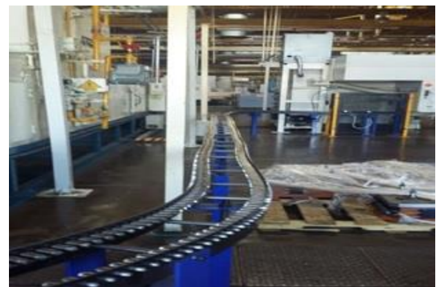
Figure 7 Conveyor Belt Installation Source: Prepared by the authors
