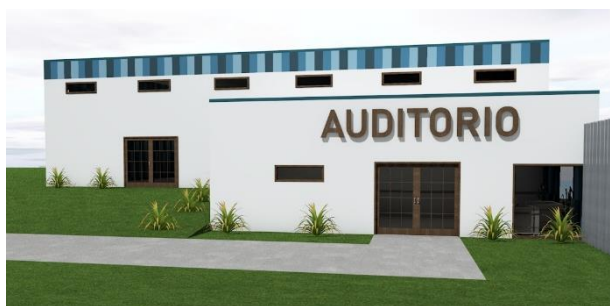
Figure 15 Main façade of building 2 Source: (Díaz, 2021)
