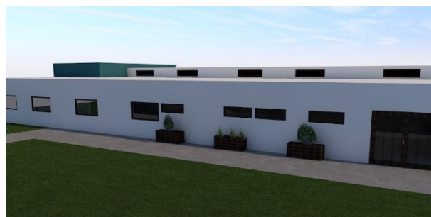
Figure 14 Side facade of building 2 Source: (Díaz, 2021)
