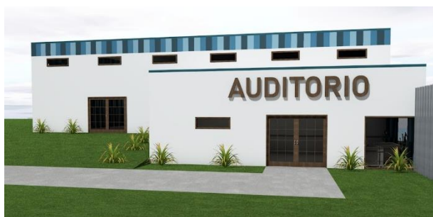
Figure 15 Main façade of building 2 Source: (Díaz, 2021)
