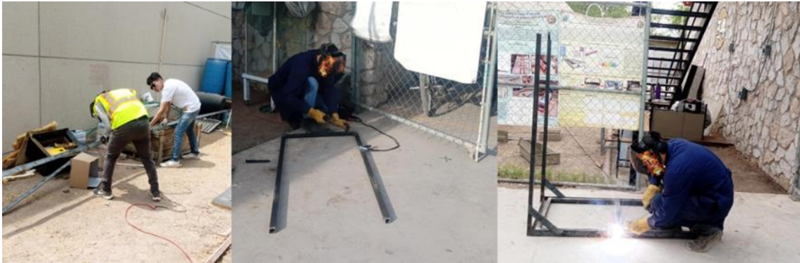
Figure 5.11 Taking of measurements and welding
