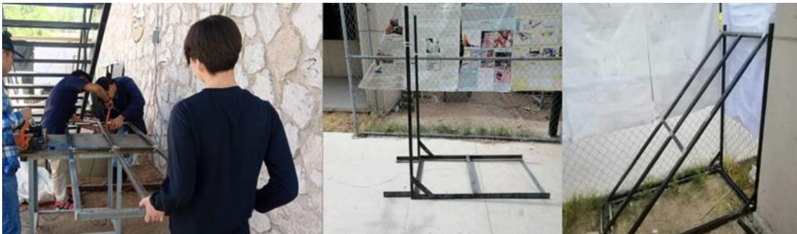
Figure 5.12 Joining the pieces
