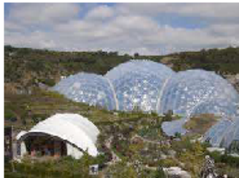
Figura 5.3 Nicholas Grimshaw Architects, Eden Project, Cornwall UK
