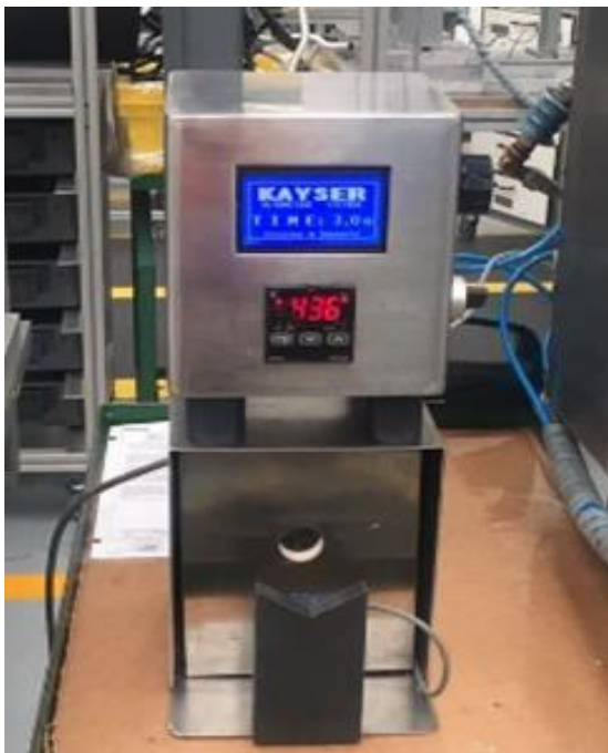
Figure 2.19 Camera installation inside the Kayser facilities
