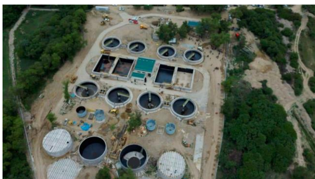
Figure 1 Photograph of the San Blas treatment plant
