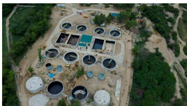
Figure 1 Photograph of the San Blas treatment plant
