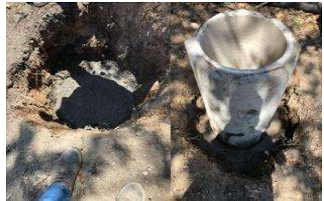
Figure 1 Tiling and placement of the concrete pipe Own Source
