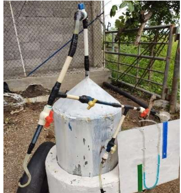
Figure 4 Floating hood biodigester prototype Own Source
