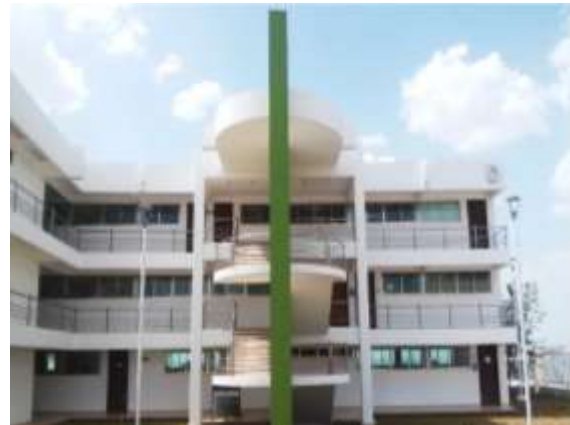
Figure 7 "D" BUILDING, Campus V Faculty of Engineering. North side Source: Own
