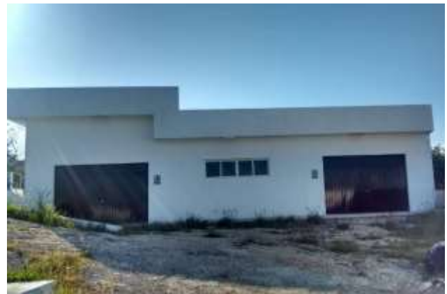
Figure 10 LABORATORY OF STRUCTURES, Campus V Faculty of Engineering. Southwest side Source: Own
