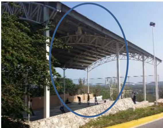
Figure 11 MULTIPLE USES COURSE, Campus V Faculty of Engineering Source: Own
