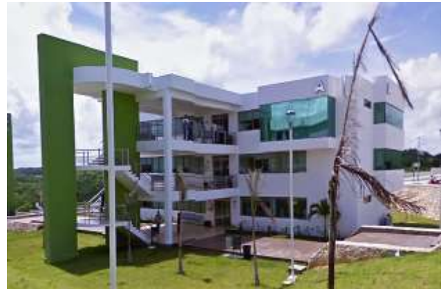
Figure 5 BUILDING "A", Campus V Faculty of Engineering. Southeast side Source: Own
