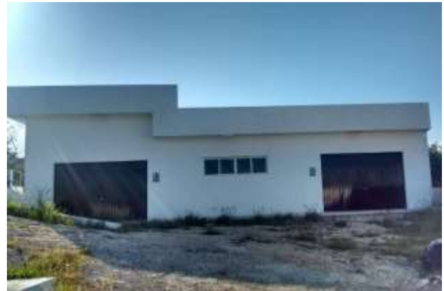
Figure 10 LABORATORY OF STRUCTURES, Campus V Faculty of Engineering. Southwest side Source: Own
