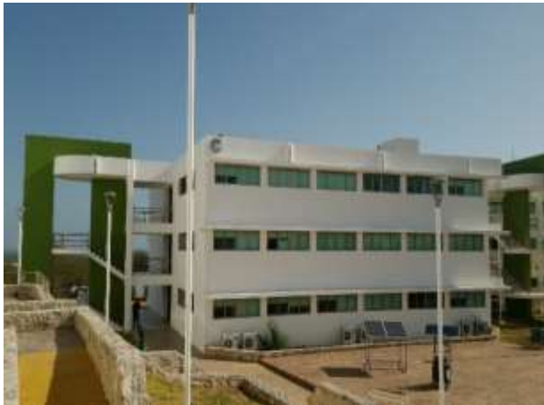
Figure 6 "C" BUILDING, Campus V Faculty of Engineering. North side Source: Own
